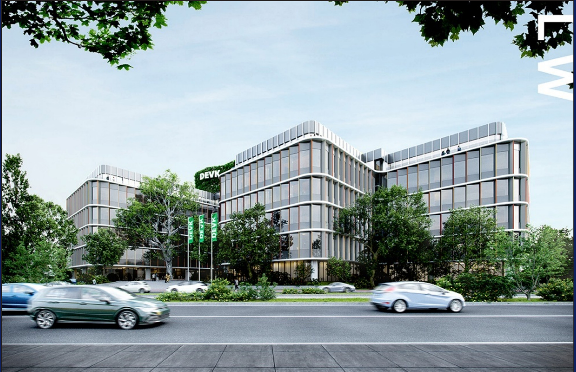
The DEVK headquarters after energy-efficient refurbishment. © Lengfeld & Wilisch Architekten PartG mbB ZWP INGENIEUR AG, GERMANY
